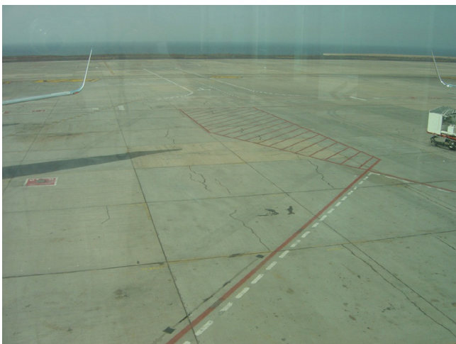
Fig. 1. Cracks in an airport apron – Airport Santa Cruz de Tenerife (photo. K. Falkowski).
