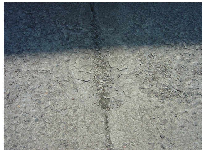
Fig. 2. The loss of the upper layer of concrete after a 20-year usage period (photo. K. Falkowski).
